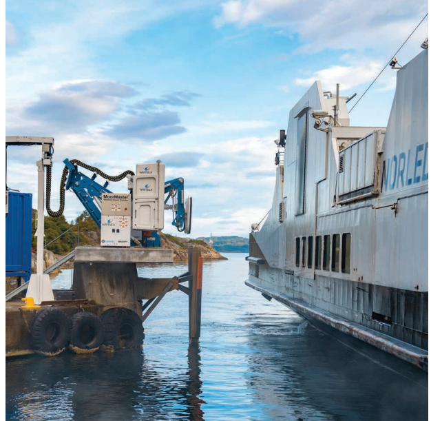
Figure 13. The Wärtsilä inductive charging system for charging the MF Folgefonn. (Source: Wärtsilä; used with permission.)
