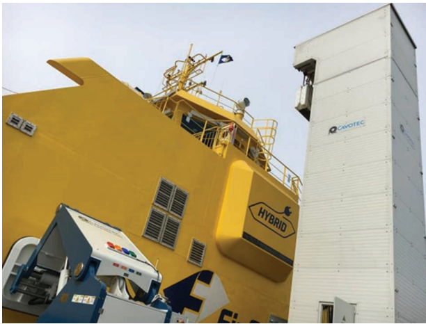
Figure 8. The Cavotec Automated Plug-in System tower used for charging the MF Elektra . (Source: Cavotec; used with permission.)
